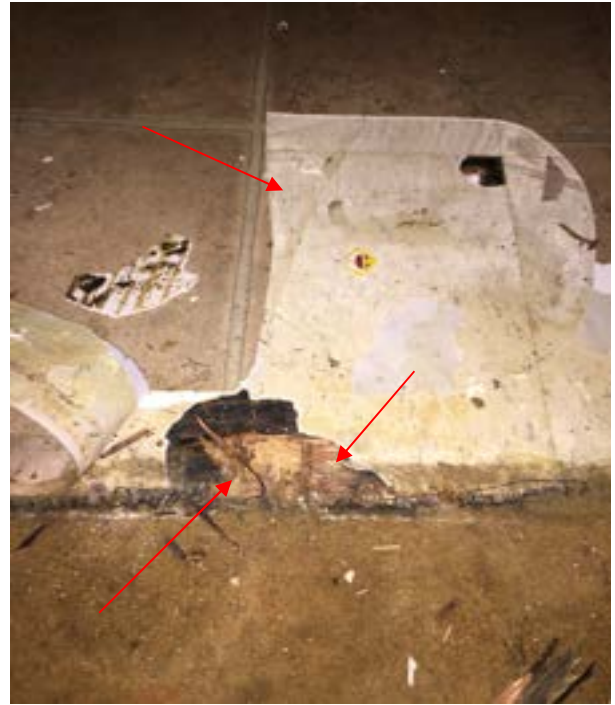
PHOTO No. 6 Typical View of Positive Black Mastic Below the Layers of Flooring. Top: Brown Linoleum, Second Layer White Floor Tile, Third Layer Plywood, Fourth Layer Floor Tile and Black Mastic
